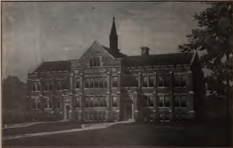
St. Mary's School, Marion, O. Wilbur T. Mills, Architect, Columbus, O.
